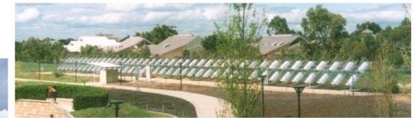
TAFE/Murdoch Rockingham – 250kW Mirror-concentrated PV system - Campus Energy Demand 50% Carbon-free
